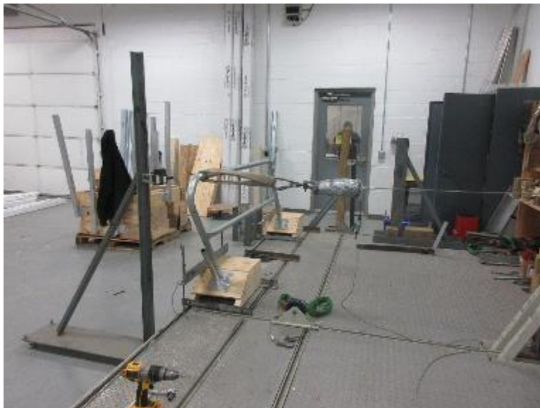
Photo No. 5 Concentrated Horizontal Load at End of Top Rail
